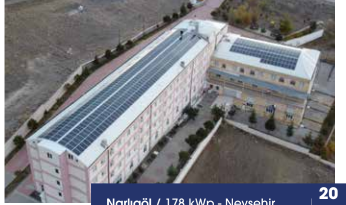
Narlıgöl / 178 kWp - Nevşehir
