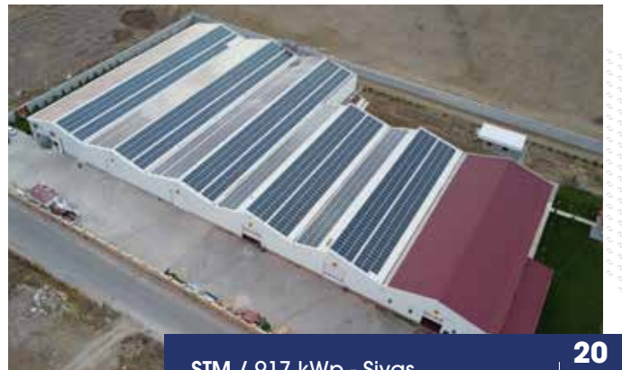
STM / 917 kWp - Sivas
